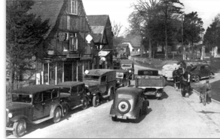
South Cambs Electrical Motor Company in Station Road
